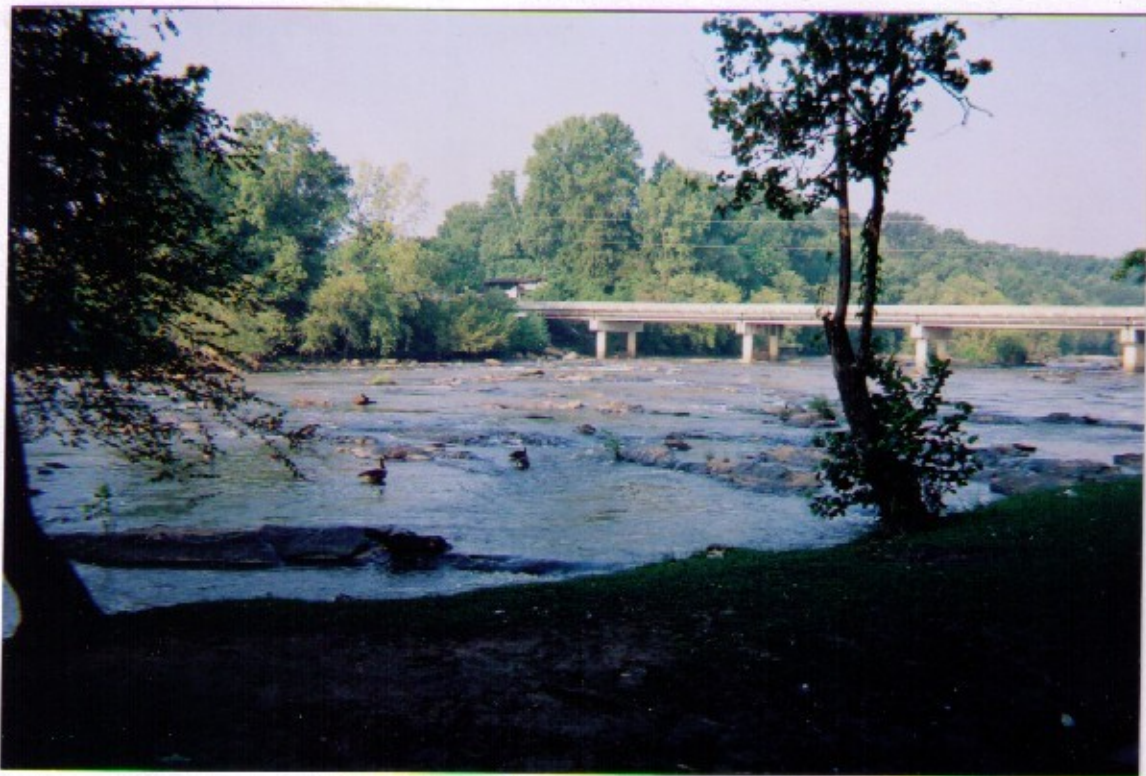
Shoals on the Saluda River at Ware Shoals, S.C. about 3 mi from Turkey Creek Baptist Church.
