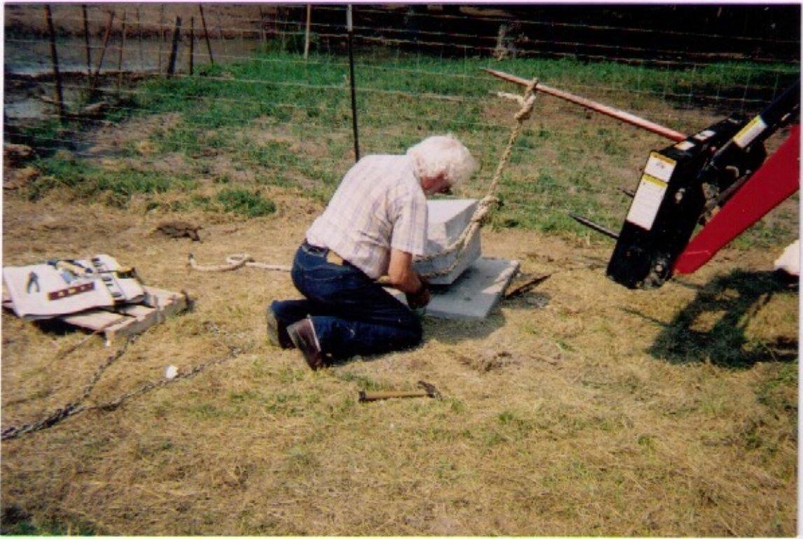
Fritz Elmhorst helping Alton level the base.
