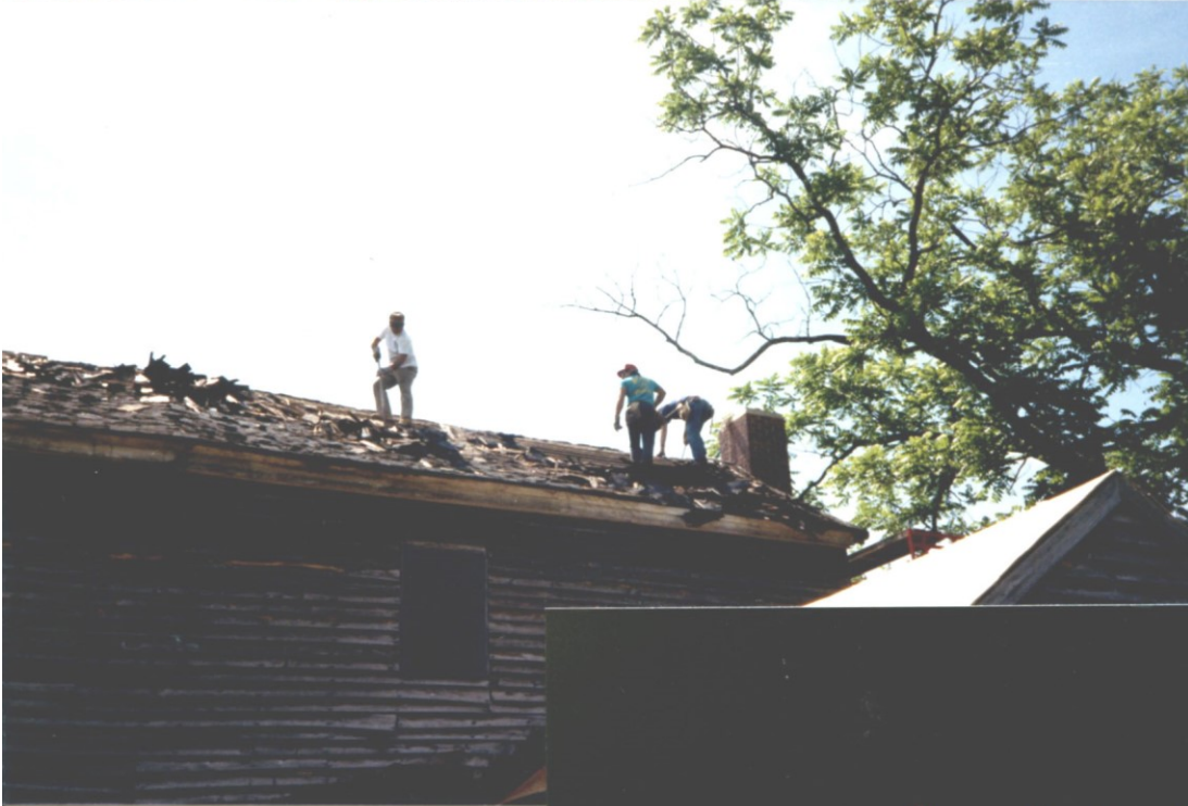
Above: Guy, Dale and Nathan removing the old roofing from the Obediah house.
